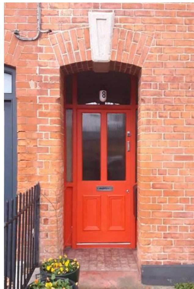
No.8 – Repair of Historic Door - 2021
