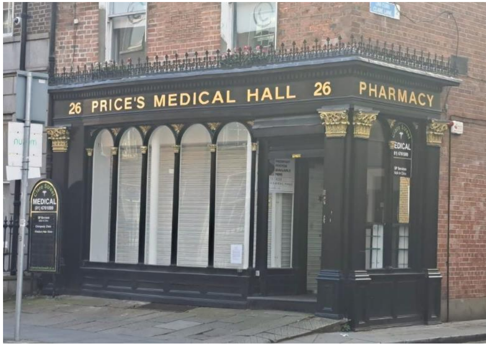
Repair of Victorian shopfront – BHIS 2020 & HSF funding 2021
