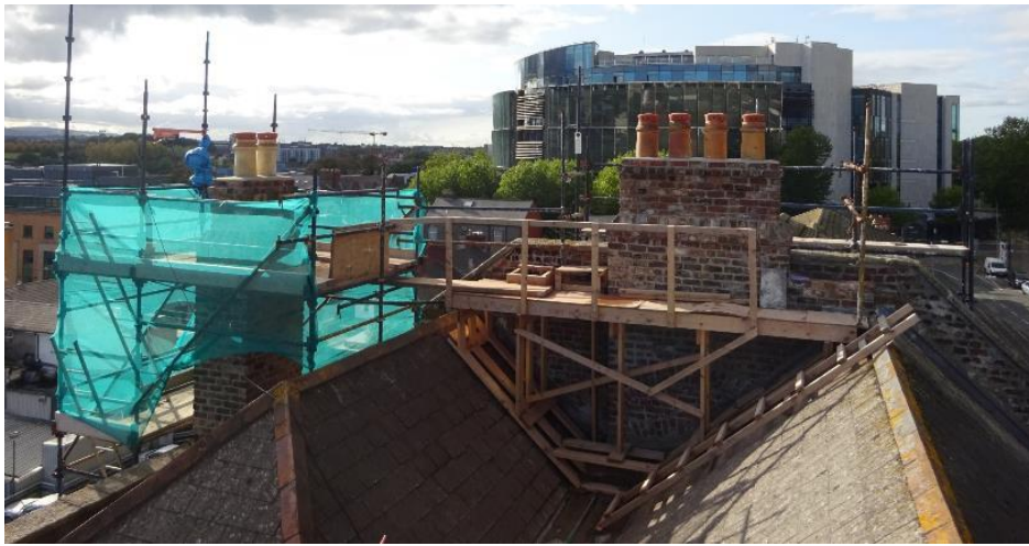
Chimneystacks & Roof Repair 2020
